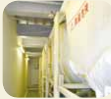
We have six 20t large cloth silos and six 750kg small cloth silos.
